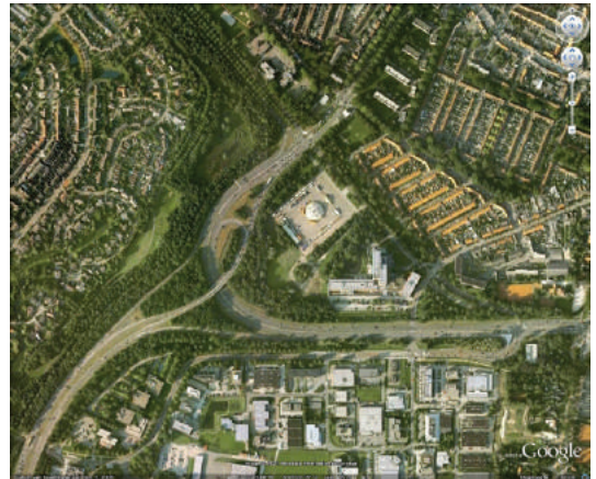
aerial photograph of existing situation
