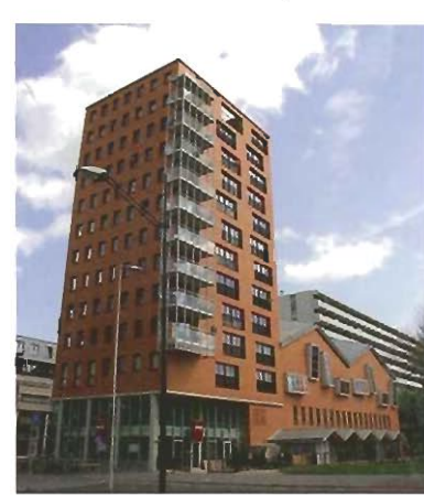
19 DE KANDELAAR MULTIFUNCTIONAL BUILDING (2005–2007) Architects: Ria Smit Address: Bijlmerdreef 1239
