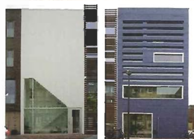
7 PRIVATE HOUSES (2004–2008) Architects (clockwise starting top left): Diederendirix, VMX, FARO Architecten, Rocha Tombal Architecten Address: Jan Olphert Vaillantlaan, Cornelis Zillesenlaan
