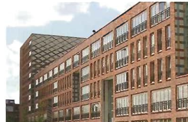
16 GERENSTEIN APARTMENT BUILDING (2007) Architect: Heren 5 Address: Bijlmerdreef 938–1092
