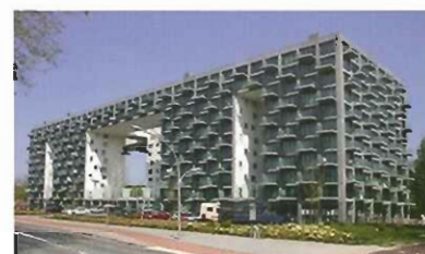
29 PARKRAND APARTMENT BUILDING (1999–2008) Architect: MVRDV Address: Dr. Collijnstraat
