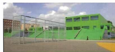
27 DE KIKKER COMMUNITY SCHOOL (2009) Architect: DOK architecten (Liesbeth van der Pol) Address: Evertswertplantsoen 3
