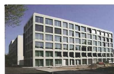
20 DISTRICT OFFICE AND HOUSING (2005–2007) Architect: Claus en Kaan Architecten Address: President Kennedylaan 923
