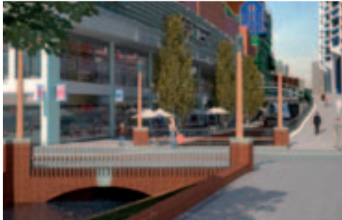
Repair of the water structure, Zaandam - PM 314
