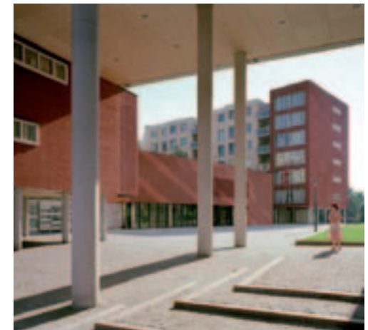
Wide entrance as point of access to the collective space, Olympisch Kwartier, Amsterdam - PM 286
